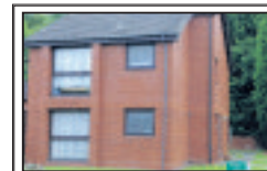
STATION ROAD OLDHILL
